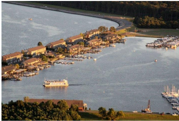
THE BREAKERS ON THE RESERVOIR
