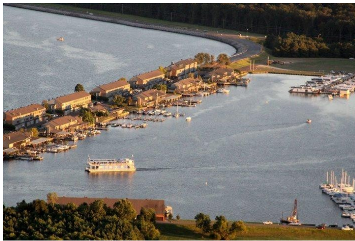
THE BREAKERS ON THE RESERVOIR
